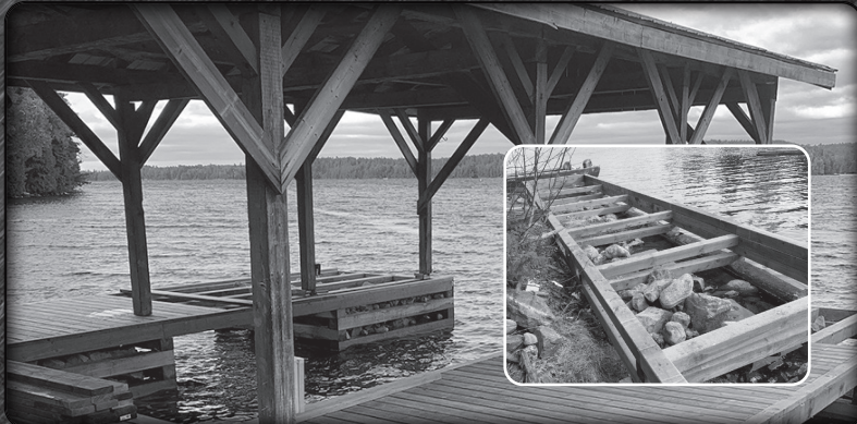
Crib and Dock Construction
