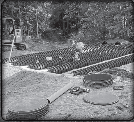
Septic System Installaton
