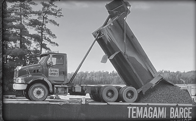
Barging Materials & Equipment
