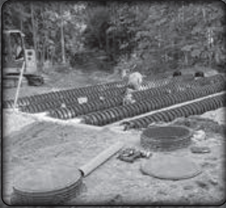
Septic System Installaton
