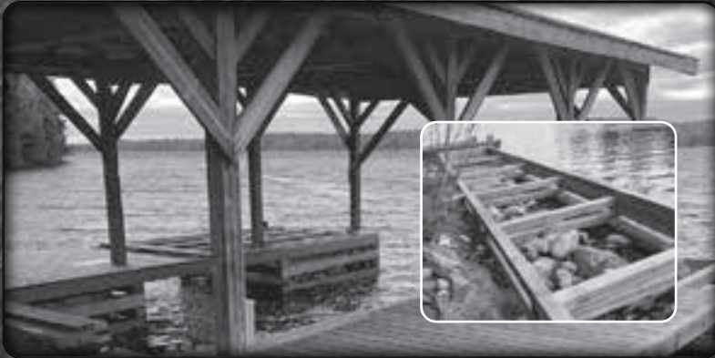
Crib and Dock Construction
