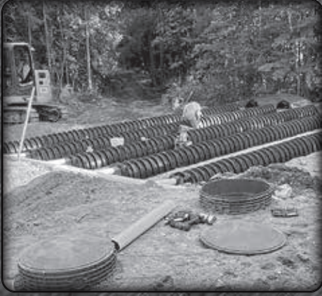
Septic System Installaton
