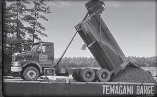
Barging Materials & Equipment
