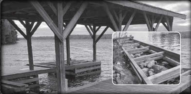
Crib and Dock Construction
