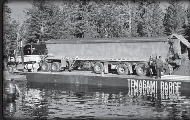
Barging Materials & Equipment
