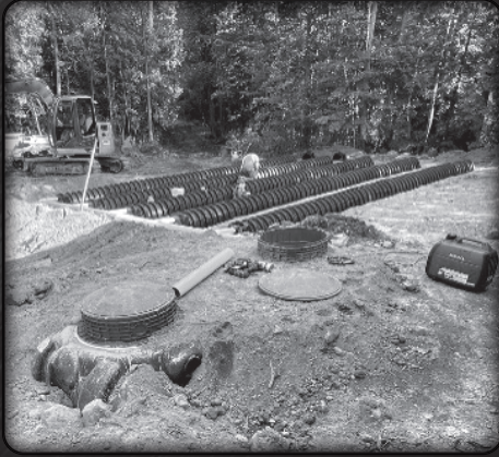
Septic System Installaton
