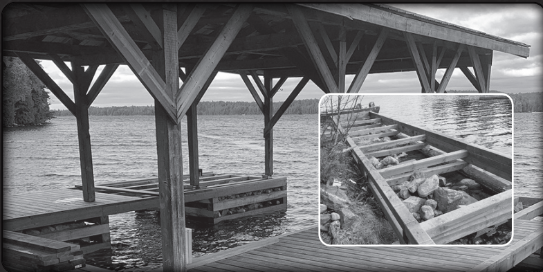
Crib and Dock Construction
