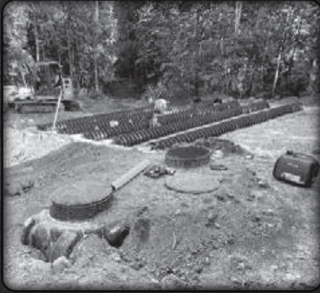
Septic System Installaton
