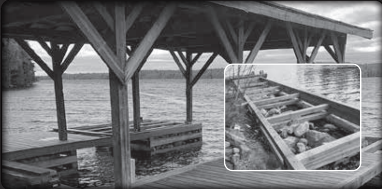
Crib and Dock Construction
