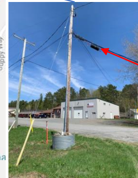
Fibre aerial enclosure
