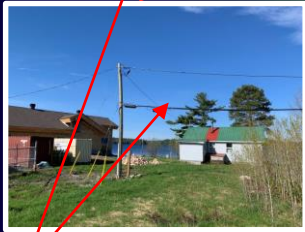
Aerial fibre optic cable
