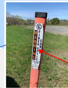
Buried fibre marker
