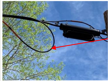
Ontera aerial fibre coil (slack cable)
