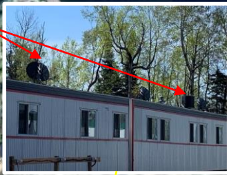
Construction trailers c/w Xplornet Internet dishes
