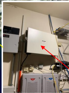
Ontera patch panel inside health centre
