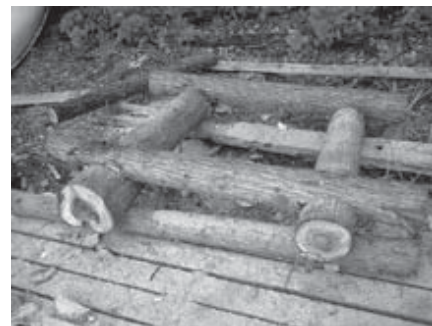
A loon nesting platform under construction. Photo by Justin Metz.
