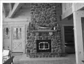
Stone Fireplaces & Repairs
