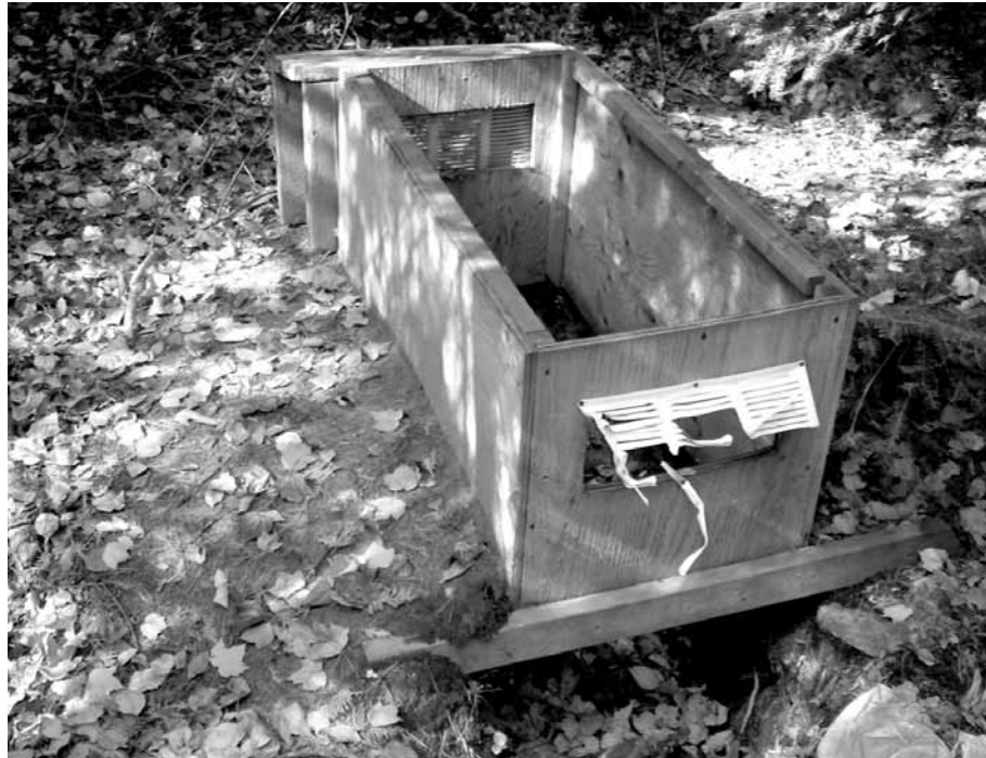
This privy at a busy campsite is in dire need of replacement. Photo by: Andrew Healy
